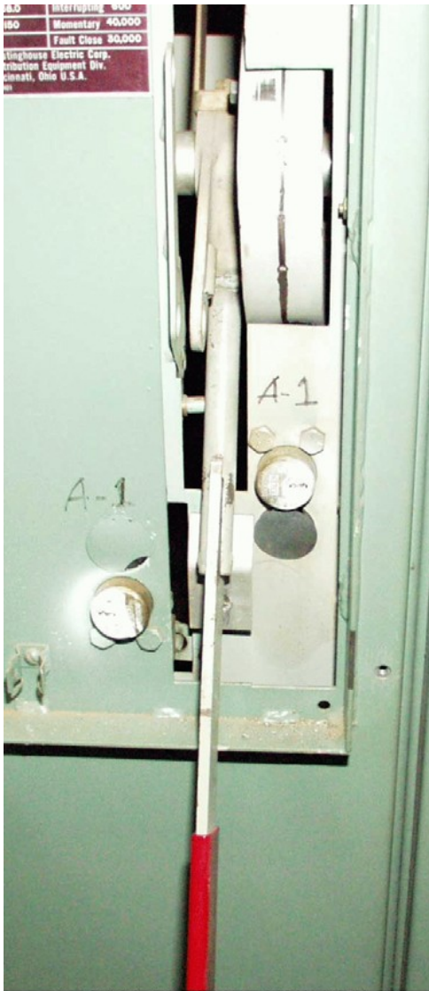
Fig. 3A WLI SWITCH IN OPEN POSITION (With non removable operating handle)
