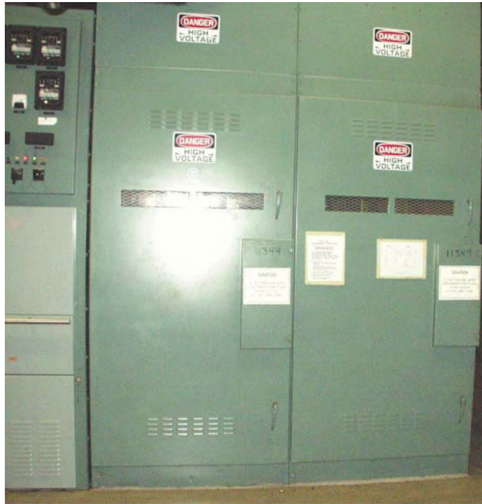
Fig. 1 WESTINGHOUSE 34.5KV LOAD INTERRUPTER SWITCH TYPE WLI
